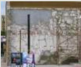
The wall at 4th & Buckeye just after stucco repair was done to close a 3" gap in the substrate.
