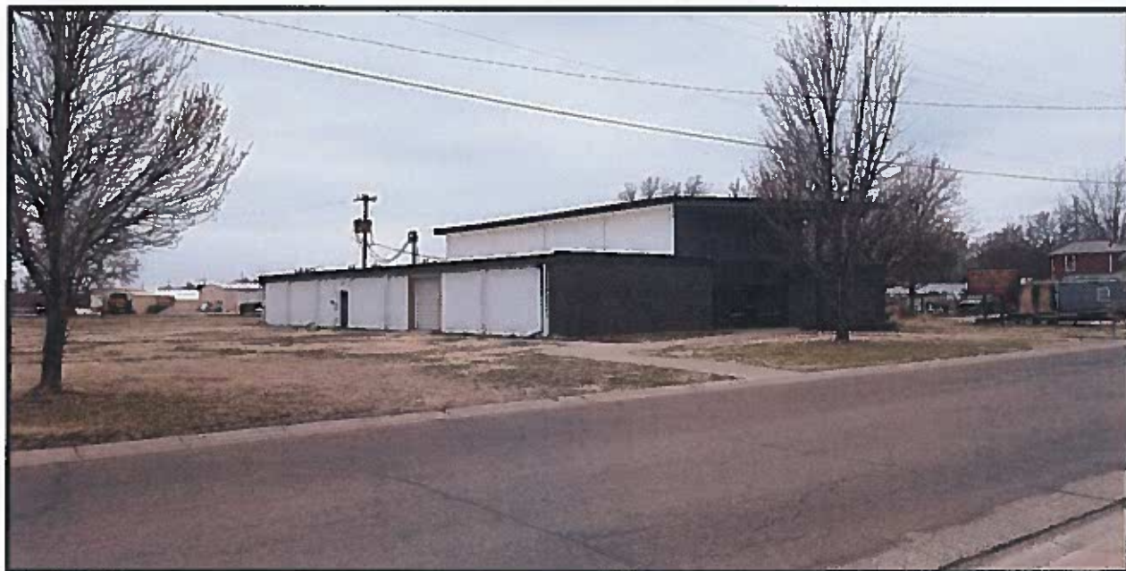
North Side of 108 SE 6 th Street
