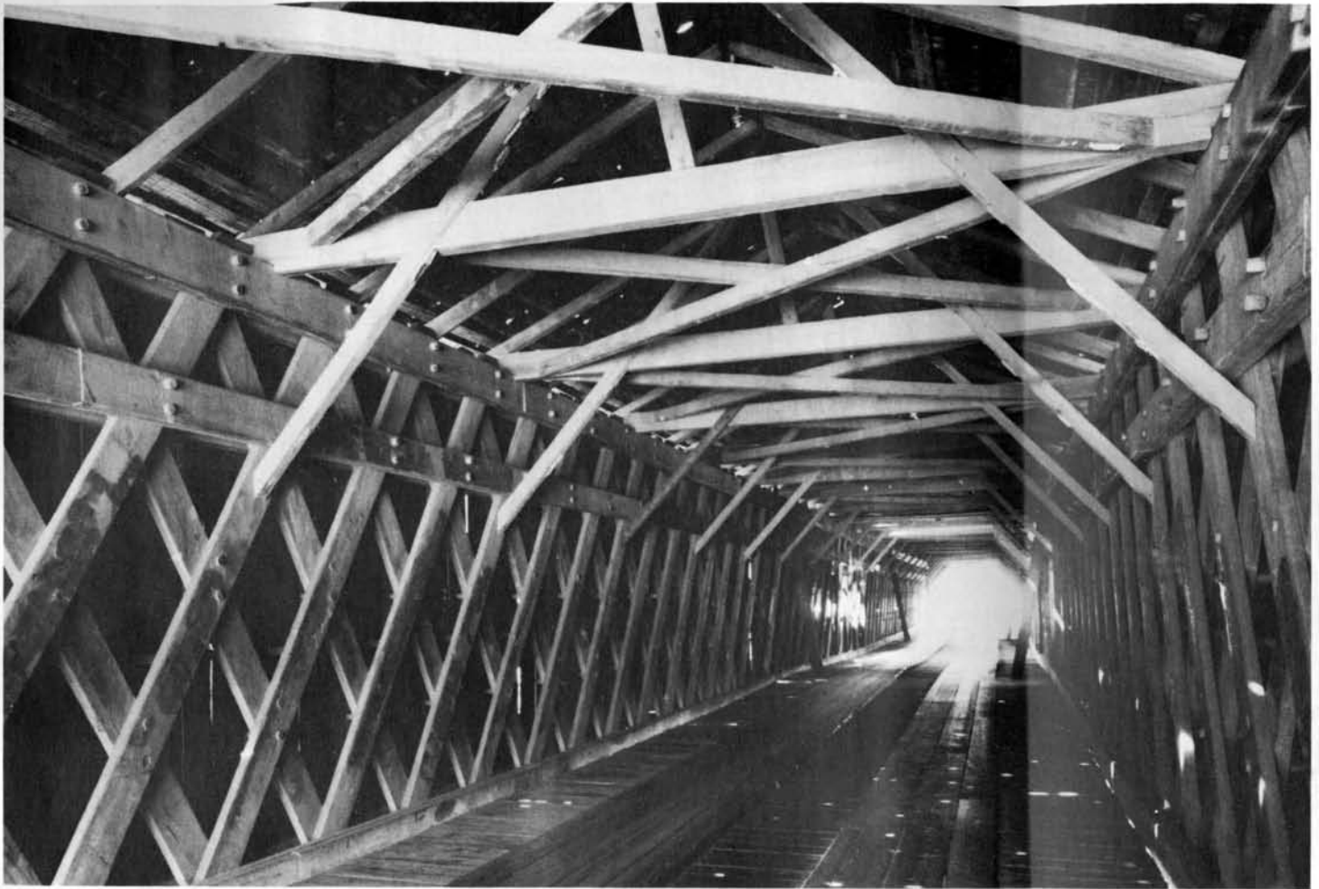
Watson Mill Covered Bridge, Comer vicinity, Oglethorpe County, Georgia. This 1885 frame bridge, an important example of the patented Town lattice truss design, has a 229 foot span over the South Fork of the Broad River, and is still in use. (Photo by: James R. Lockhart).
