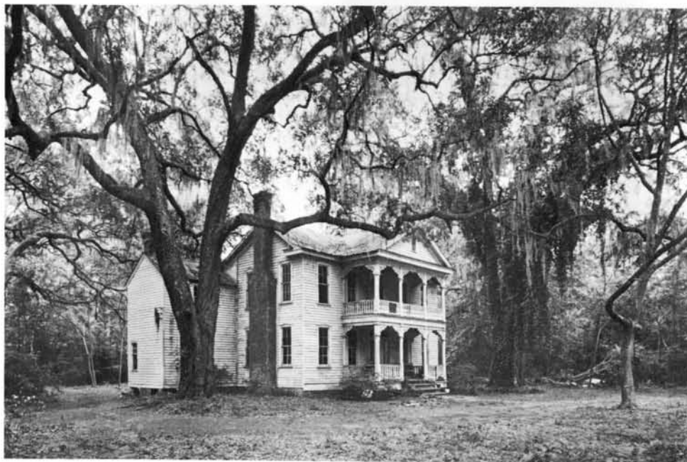
The Sylvester Mumford House, Waynesville vicinity, Brantley County, Georgia. Built c. 1848, this building is architecturally significant for illustrating changing styles in architecture as reflected in the evolution of a house. The core of the house is typical of the Plantation Plain style residence constructed in rural Georgia during the first half of the 19th century. The post-Civil War additions, particularly the front porch with its decorative scrollwork brackets and balusters and a polygonal south wing are Victorian in character and illustrate the owner's attempt to keep up with the latest in architectural styles and tastes. (Photo by: James R. Lockhart).
